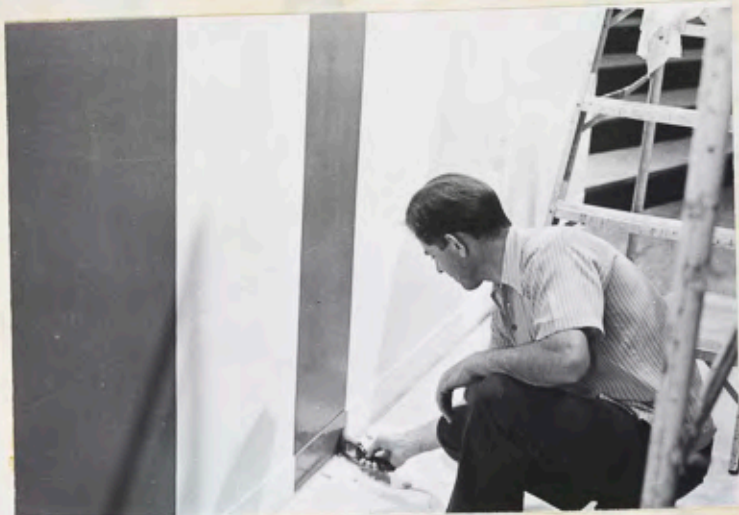
Frank doing the lines around the coverlet in the central hall.
