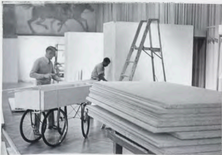
Our stuff out and the carpenters getting the construction down in the Armour Gallery.
